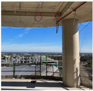
Quins Debris Containment Netting is designed to wrap around buildings, particular installs with threaded M10 inserts, enabling installers to easily attach M10 eye nuts and secure the 5mm wire.
